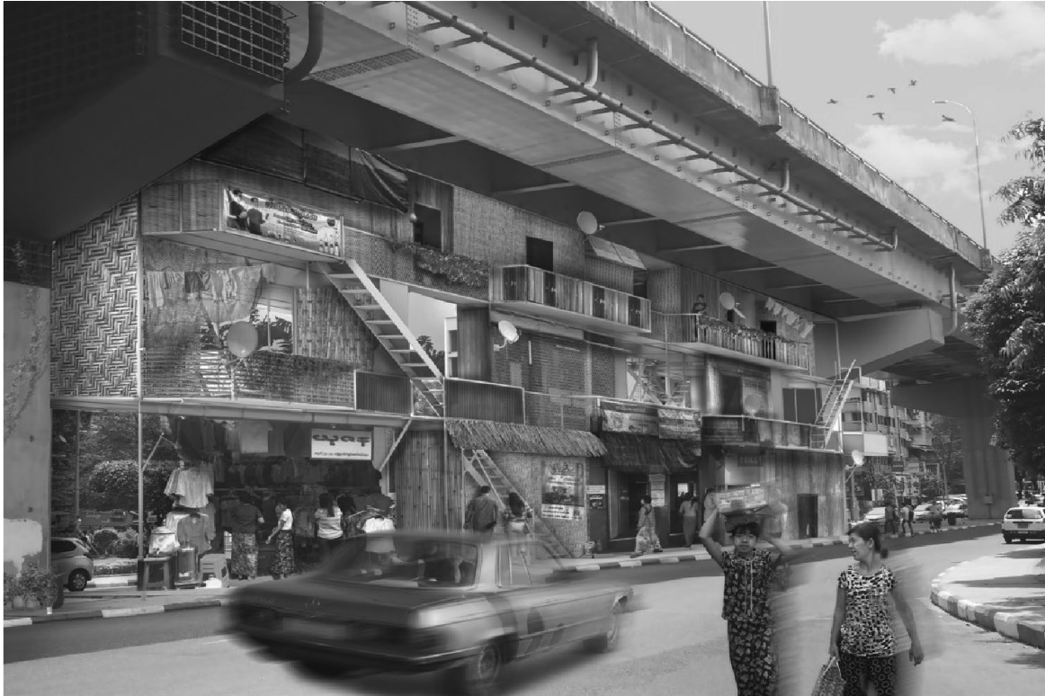
Figure 2. This project proposes to enable and empower underserved populations by leveraging existing infrastructure to benefit self builders and marginalized populations; Noah Smith, Stephen Smith, Erica Young
